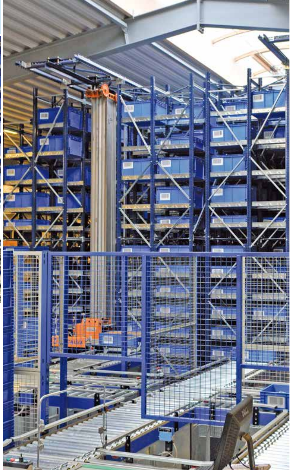
Warehouse with double depth
