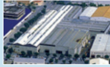
Plant in Cornellà (Barcelona), Spain
