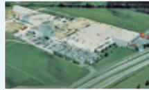
Plant in Pontiac, USA
