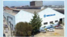
Plant in Buenos Aires, Argentina
