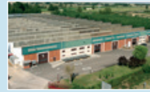
Plant in Palencia, Spain
