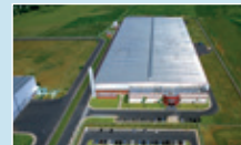
Plant in São Paulo, Brazil
