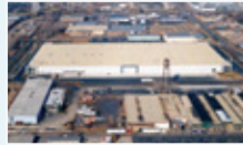
Plant in Chicago, USA
